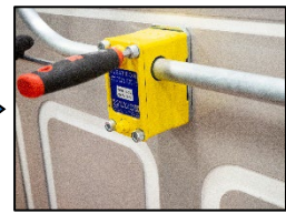
4. Loosen the screws on the siphon block...
