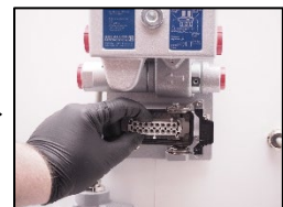
16. Check all leaders in the main socket. If bad conditions – replace the connection socket!
