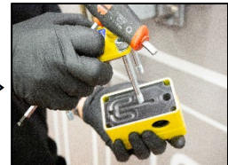
8. Take of the cover of the siphon block.
