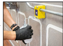
16. Pump in the oil.
